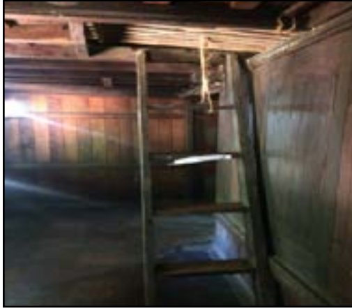
Figure No.13: Soldara entrance, Eka Sālā, Tivandrum
